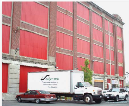
Davico has moved to a 32,000-square-foot facility that used to house a major department store.
